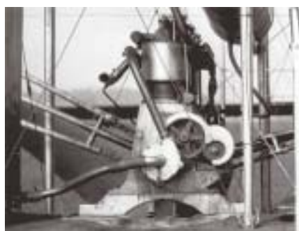
1910 Wright Vertical Four Engine
